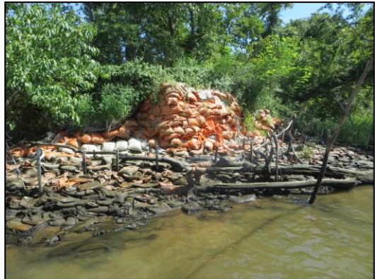
Sandbagging protecting a prehistoric site along a river in Queen Anne's County.
